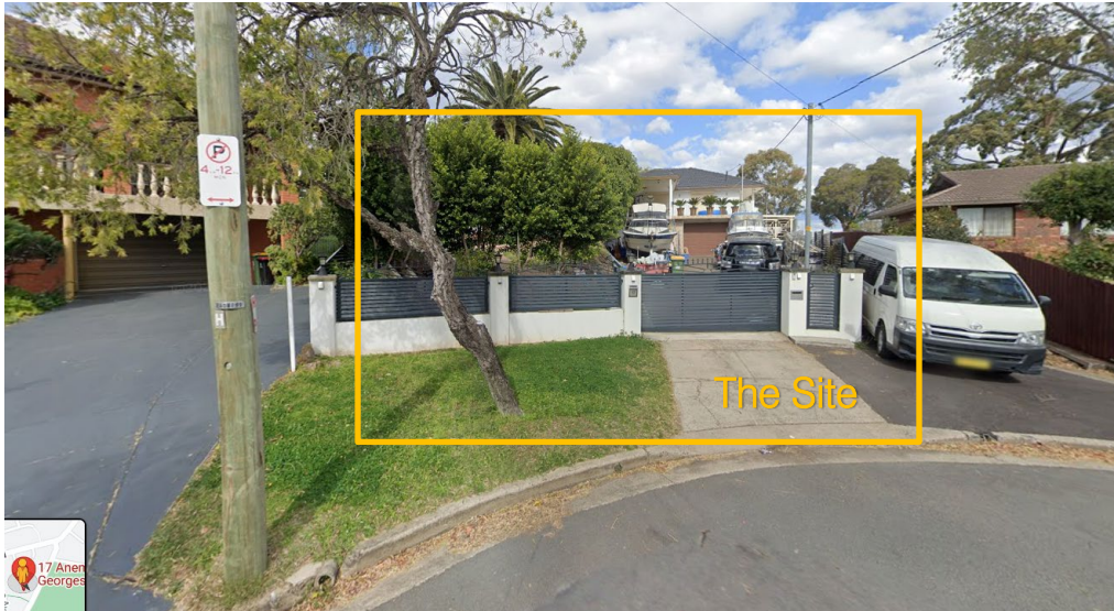
Figure 2: View to the existing dwelling house, as seen from Anembo Avenue. (Source: Google Map)
